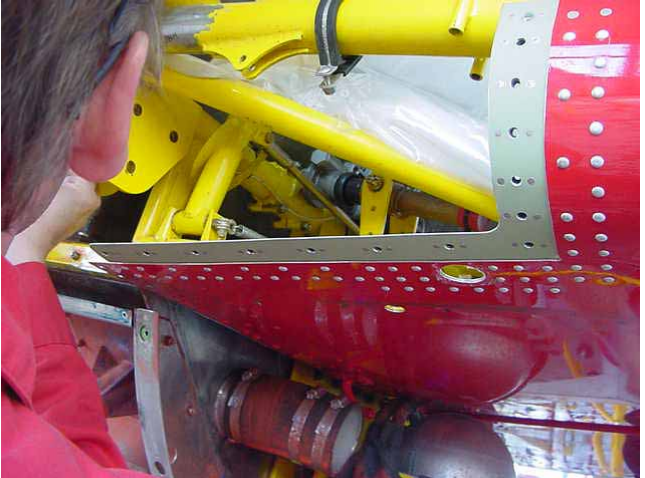
Image #4 Access panel installed.
