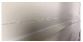
Condition 2 - Corrosion is visible around the stiffener, and the stiffener will need to be removed for replacement and for closer inspection of the skin.
