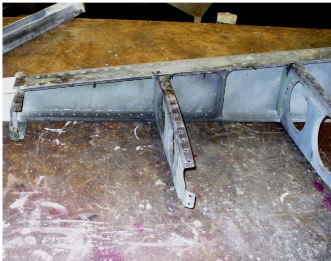
Pylon before repair
